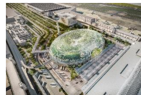
Gambar 1. Changi Airport Singapore (Sumber: Archdaily, 2019)
