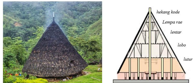
Figure 7 Mbaru niang at Wae Rebo Village, Manggarai
