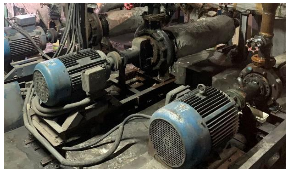
Figure 1. EBARA 65x50 FSS4JA Centrifugal Pump.
